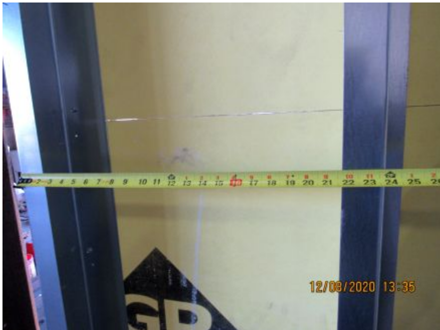
Photo No. 10 Z-girt spacing
