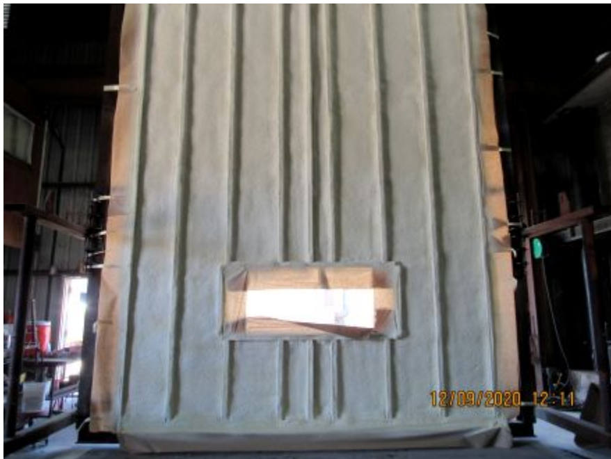
Photo No. 14 Spray foam complete
