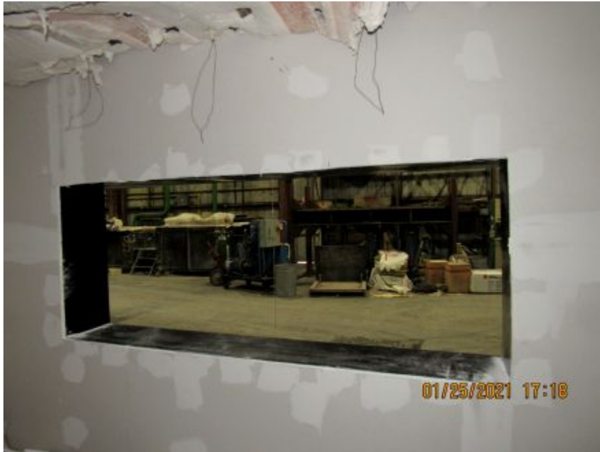
Photo No. 19 Wall interior
