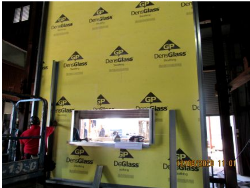
Photo No. 8 Installation of Z-girts
