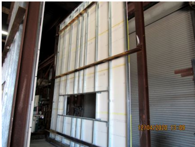
Photo No. 2 Exterior sheathing installed
