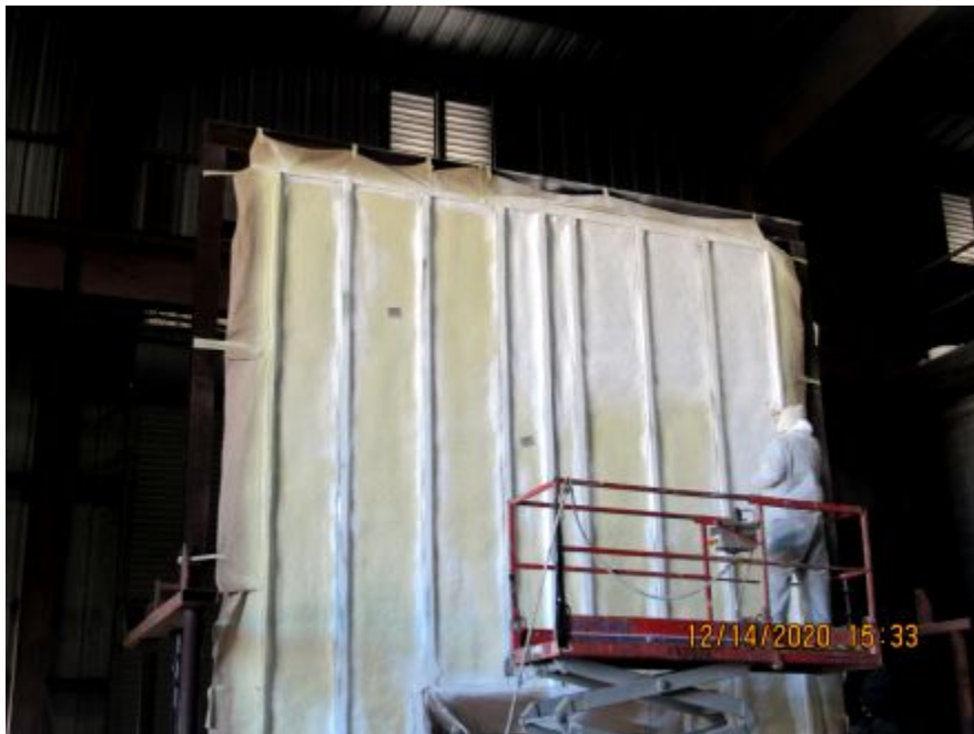
Photo No. 16 Spraying DC315
