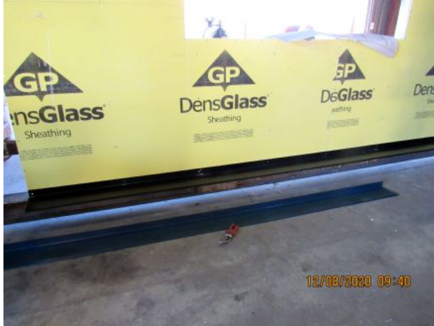
Photo No. 7 Bottom flashing installed
