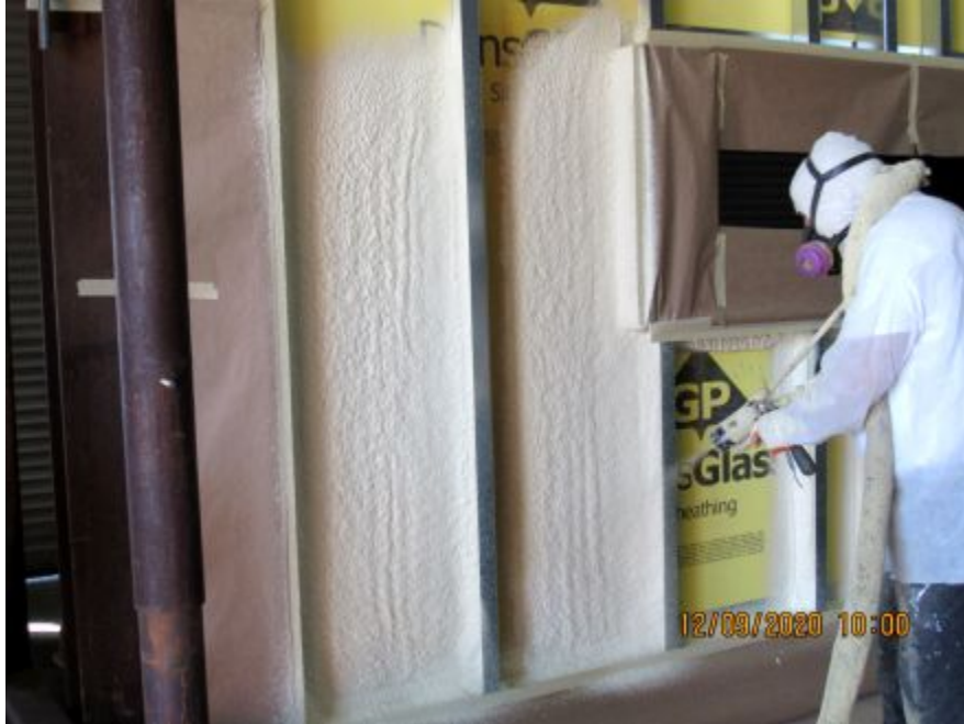
Photo No. 13 Application of spray foam
