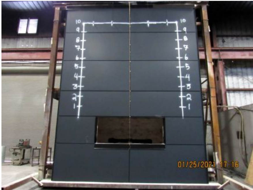
Photo No. 18 Wall assembly complete
