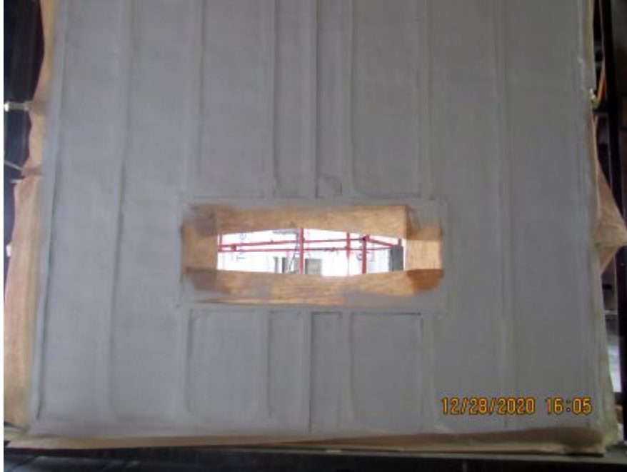
Photo No. 17 Spray complete
