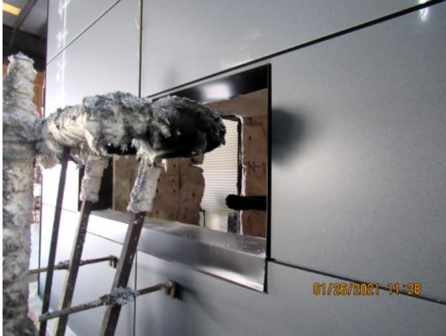
Photo No. 21 Window opening pre-test
