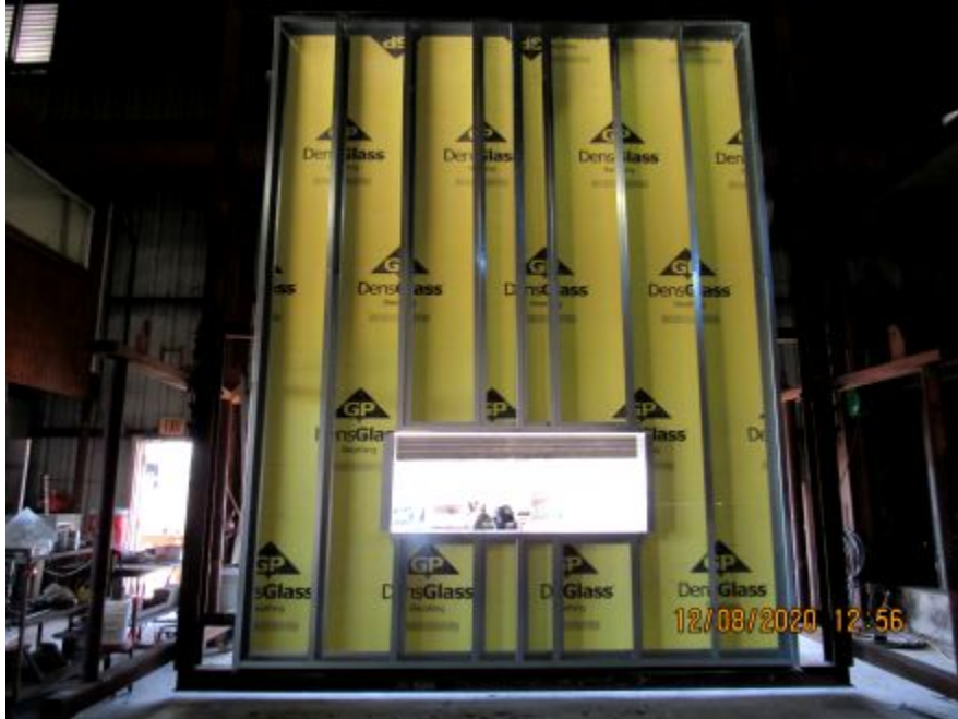
Photo No. 9 Vertical Z-girts installed
