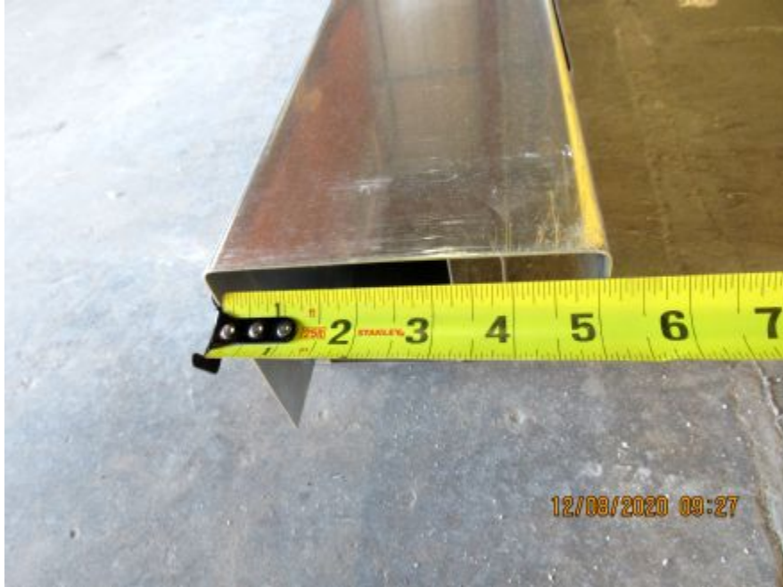
Photo No. 5 J-channel depth
