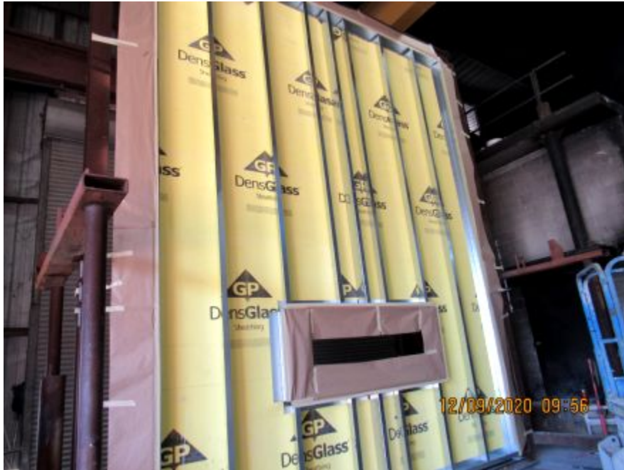
Photo No. 11 Wall pre-foam spray
